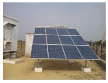
SPV based Green solutions at sites in power starved UP(E) circle. The project is approved under the Jawaharlal Nehru National Solar Mission (JNNSM) of the Government of India. We have installed 10 KW Solar Photovoltaic system for providing
